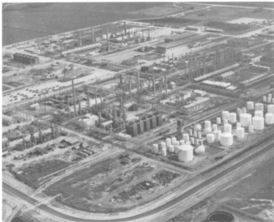
Figure 2-1. Petrochemical plant complex. (Shell Chemical.)
