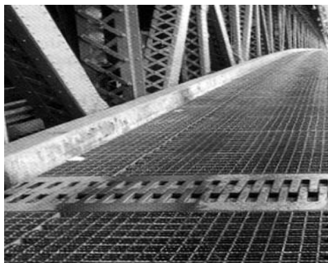
(b) Bridge expansion joint
